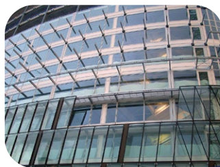
Photograph of One Angel Square (Manchester) with a double-skin façade. The building features an outer glass skin and an inner façade, forming a ventilated cavity in between. Automated louvers and operable windows in the outer skin open based on weather data, allowing air to flow into the cavity for natural cooling and exhaust [Wikipedia]
