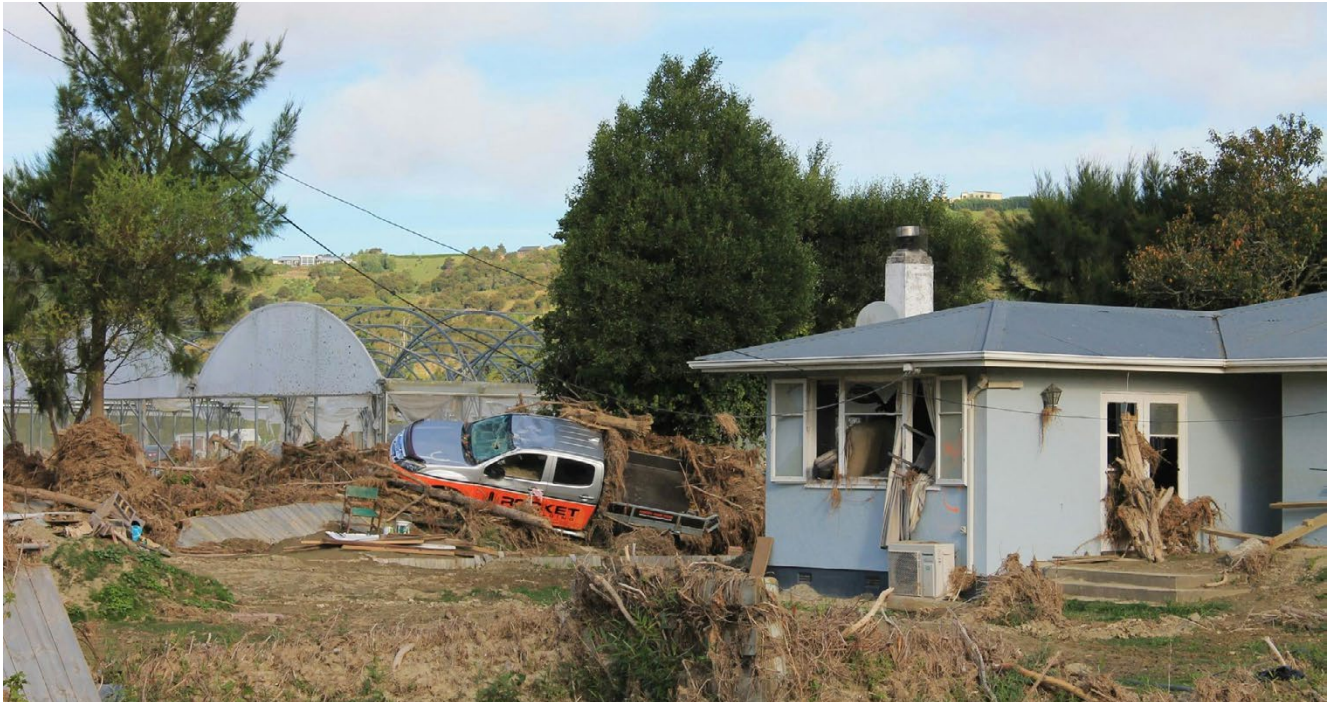
Residential property damage following Cyclone Gabrielle, Eskdale, Hawke's Bay, February 2023.
