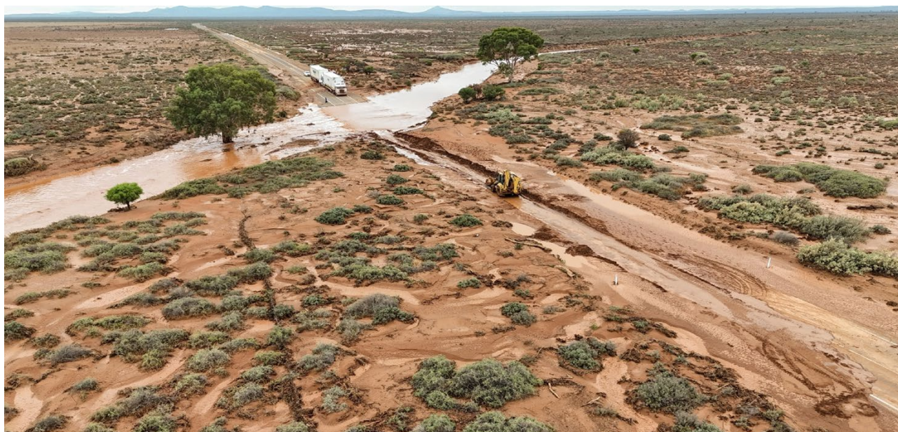
Aerial imagery captured by SASES RPA pilot of the Willochra Creek flooding impacts and attempts to clear the silt over road.
